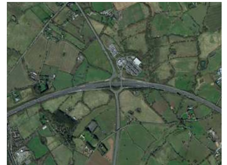
M42 Junction 2 Redditch
