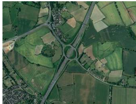
M5 Junction 7 Worcester South
